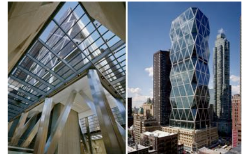
Hearst Tower NYC is LEED Platinum reducing total energy consumption by 40%, total waste to landfills by 82%, composting 100% of its wet food waste, has 100% use of reclaimed non-potable rainwater for landscaping, & reduced water use by more than 30%.
